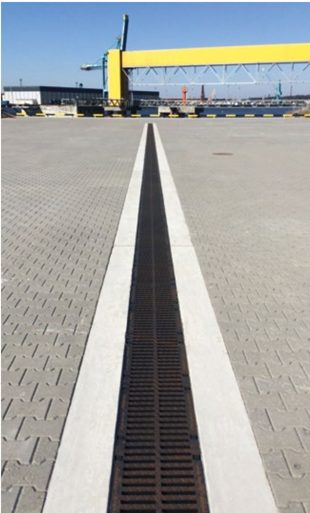
Container terminal and port, Latvia
