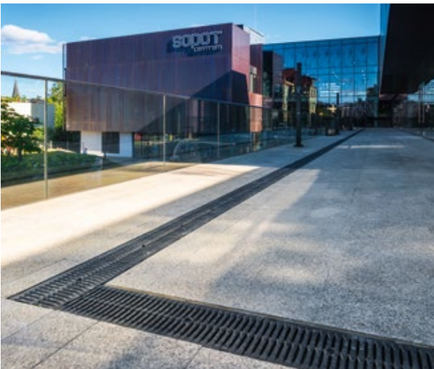
Railway station in Sopot, Poland
